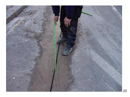
Figure 3: Picture of the microduct laying operation
